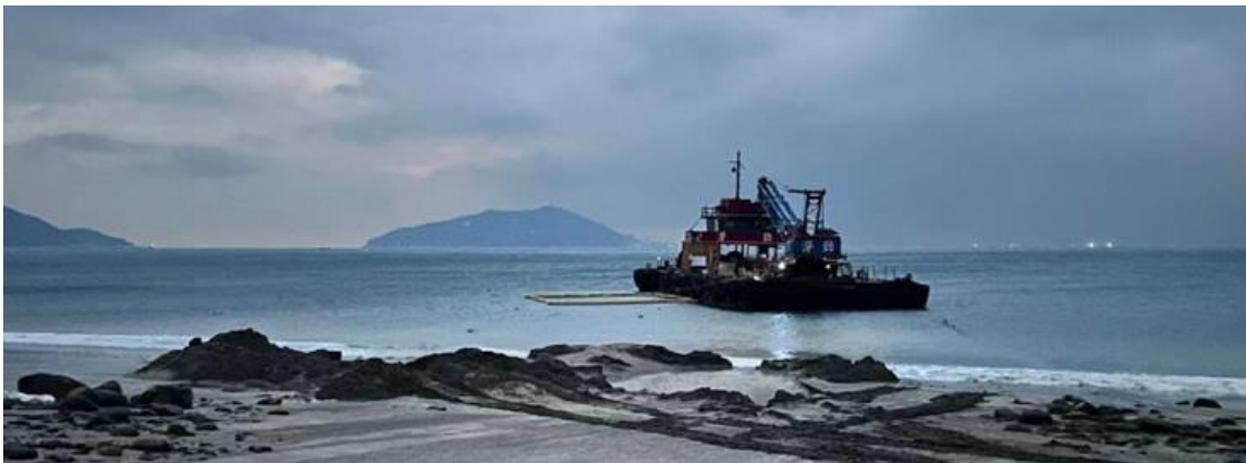
Photo 2 Photo of silt curtain setup taken on 16 Dec 2023
