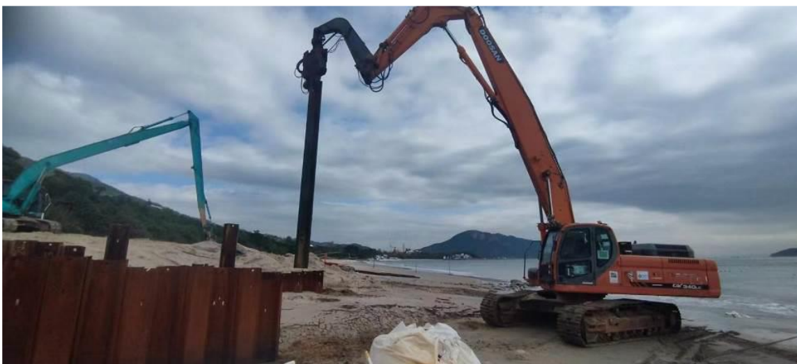
Photo 3 Photo of sheet pile removal works taken on 16 Dec 2023
