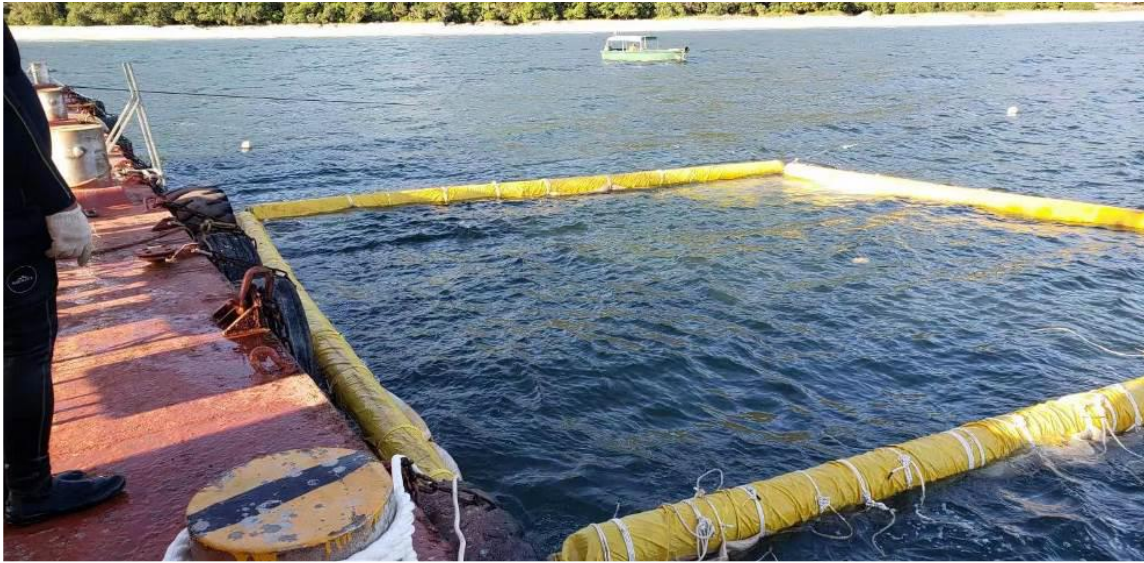
Photo 1 Hand jetting within cage type silt curtain as mitigation measure taken on 8 Dec 2023
